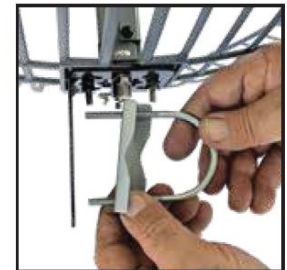
8) Depending on your mount location. You can slide assembled antenna over mast or secure U-bolts around mast on this step.
